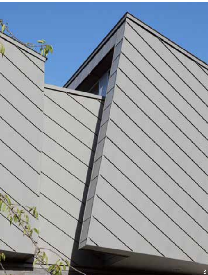
1: Benedictus school, Gent (Belgium) - Architect: Danny Vandewalle, Corijn en Leyman - Technique: VMZINC® Sinus profile. 2: Apartment House Piasek, Wrocław (Poland) - Architect: Design studio +48 Dziewoński and Łukaszewicz - Technique: VMZINC® Sinus profile. 3: Reading Girls School, Reading (UK) - Architect: Integrated Design Consultants - Technique: VMZINC® Sinus profile. 4: Sede della Facoltà di Scienze Matematiche Fisiche e Naturali dell'Università Ca'Foscari - Mestre (Italia) - Architect: Studio Architetto Mar/Architect Giovanna Mar - Technique: VMZINC® Sinus profile.
